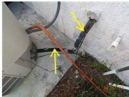
Photo 21-8 Deteriorated insulation
