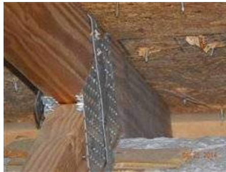
Photo 9-2 Roof to wall connection
