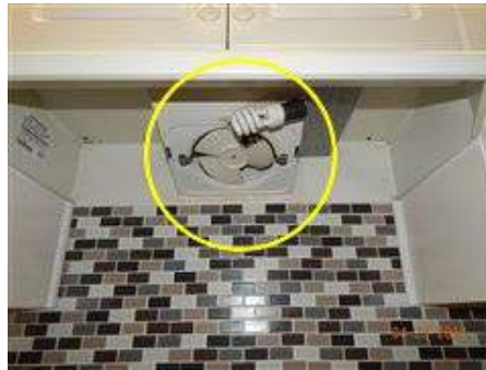
Photo 23-2 Missing filter
