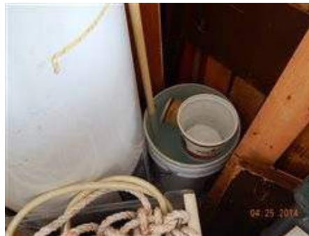
Photo 18-2 TPR drain pipe into bucket
