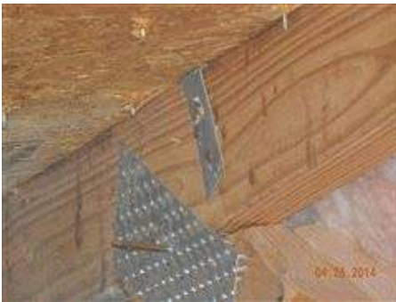
Photo 9-1 Roof to wall connection
