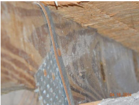
Roof to Wall Attachment
