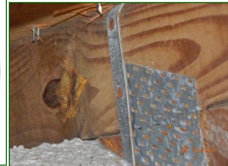
Roof to Wall Attachment
