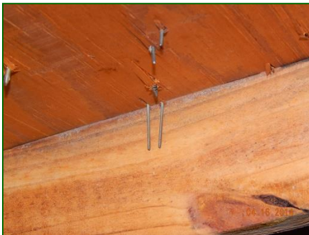
Roof Deck Attachment Staples
